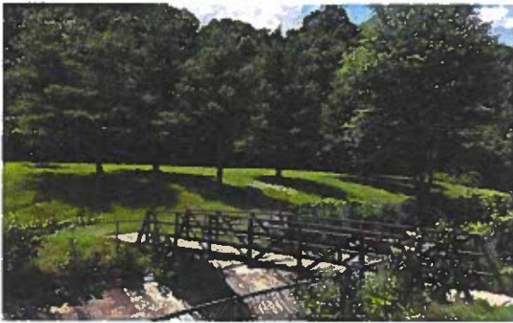
Bridge connecting Library Field and Veterans Park
