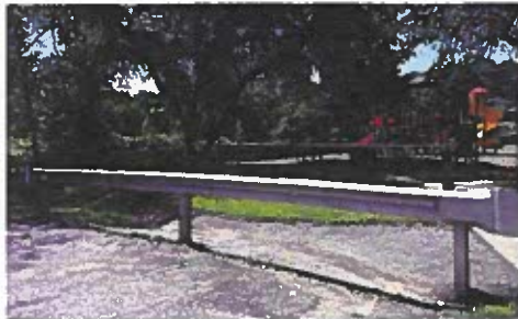
Guardrail and gutter at the front of the tot lot
