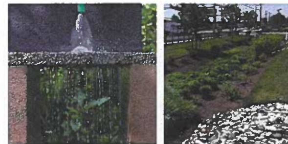
Permeable paver demonstration (left) and a rain garden in a Beltsville parking lot (right).
