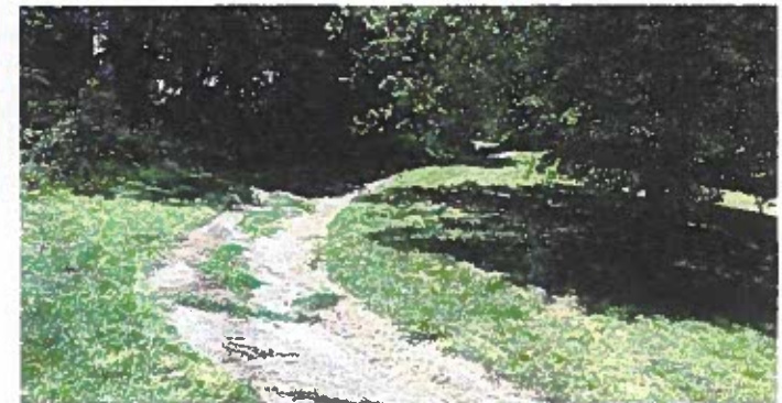
The walkway/gutter is very steep and in poor condition
