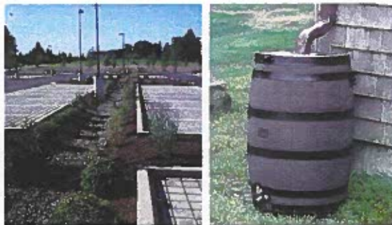
Swale in the median of a parking lot (left) and a rain barrel (right) capture runoff from impervious surfaces.
